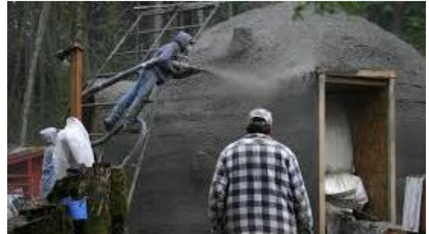
Shotcrete in Dome Construction
