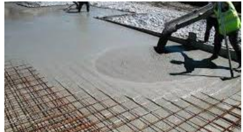
SCC in Heavy Reinforced Structure
