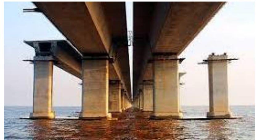
Marine Concrete Structure
